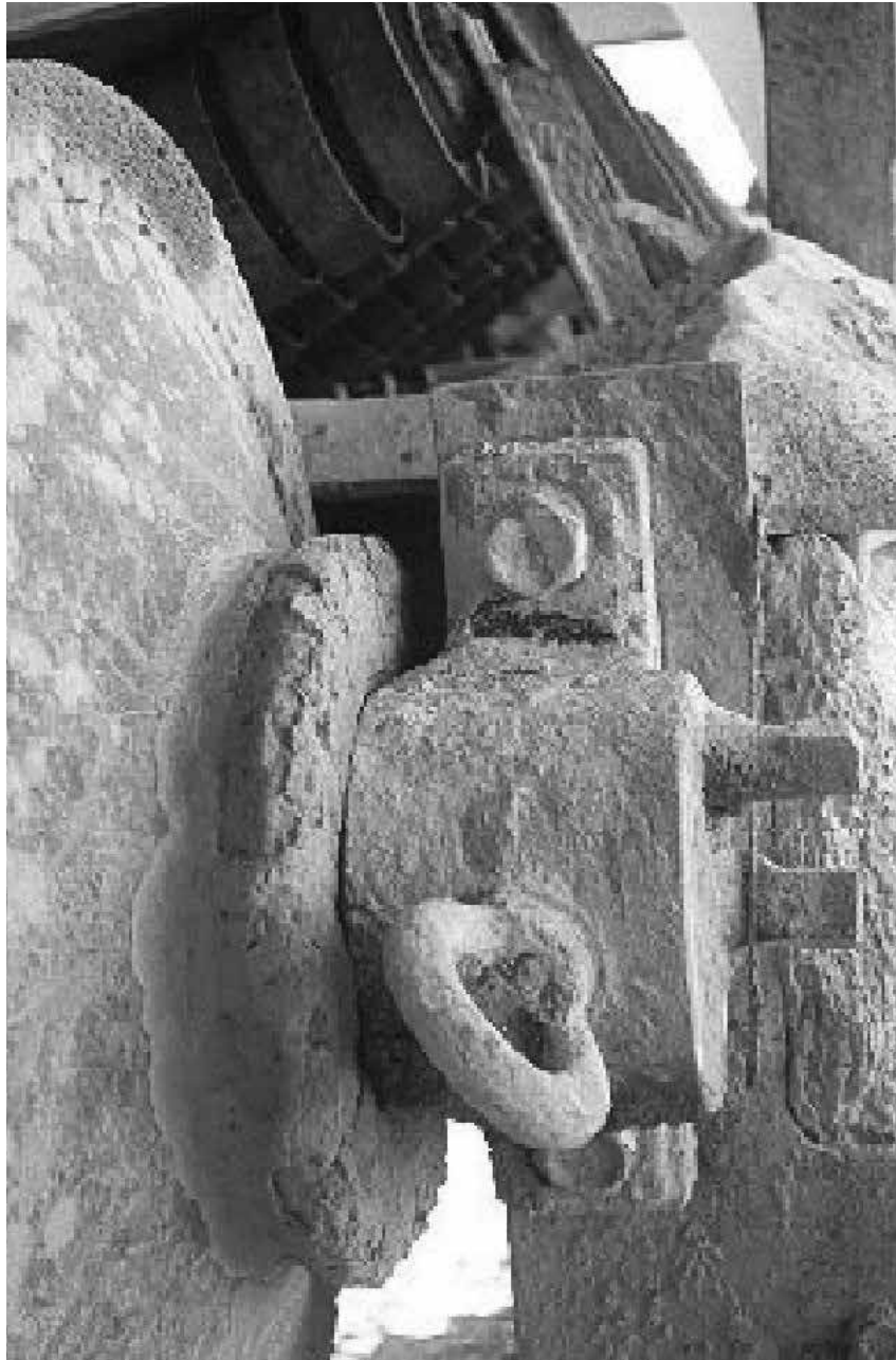
Application: Fertilizer and potash. Still in work after more than 30 years in an aggressive environment.
